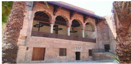
Fig.3 The summer Miqaad overlooking the inner court. After: http://archnet.org/sites/6152/media_contents/55939
