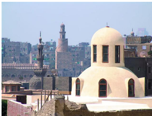
(Fig.7) The newly-constructed dome of the harem.
