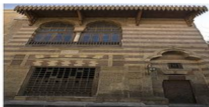
(Fig. 5) The façade of the sabil and its iron grilled window. After: ww.eternalegypt.org/
