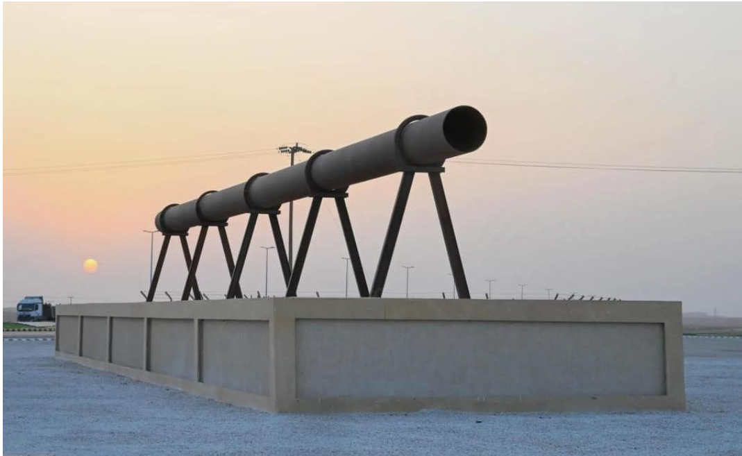
Fig. 12 The TAPLINE model located in the village of Al-Deedab east of the city of Arar, SPA
