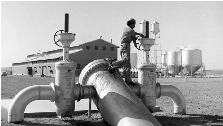
Fig. 11 Six original pumping stations were built along the TAPLINE route to pump oil, five of which are in Saudi Arabia and one in Jordan. Source: from Aramco (2021).
